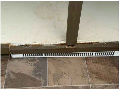
Below kitchen sink
