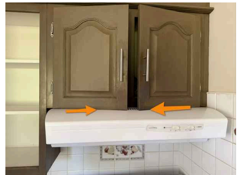
Doors rubbing on top of range hood fan
